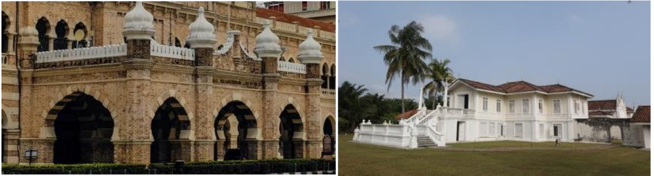
Figure 5. Color and texture of Sultan Abdul Samad Building, Kuala Lumpur and Istana Bandar Jugra, Banting
