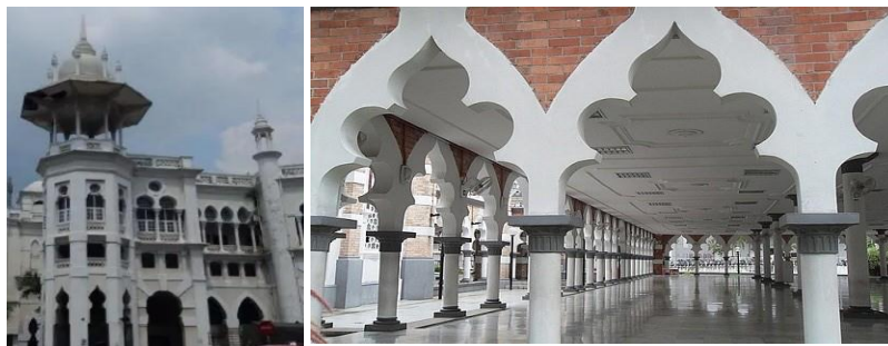
Figure 14. Pointed Mughal arches dominated along the colonnaded corridor of the building at Kuala Lumpur Railway Station Buildings and Kuala Lumpur Jamek Mosque
