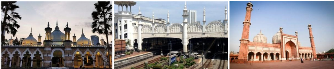
Figure 18. Turrets at Jamek Mosque, Kuala Lumpur and KTM Station Kuala Lumpur and Jama Masjid in Delhi
