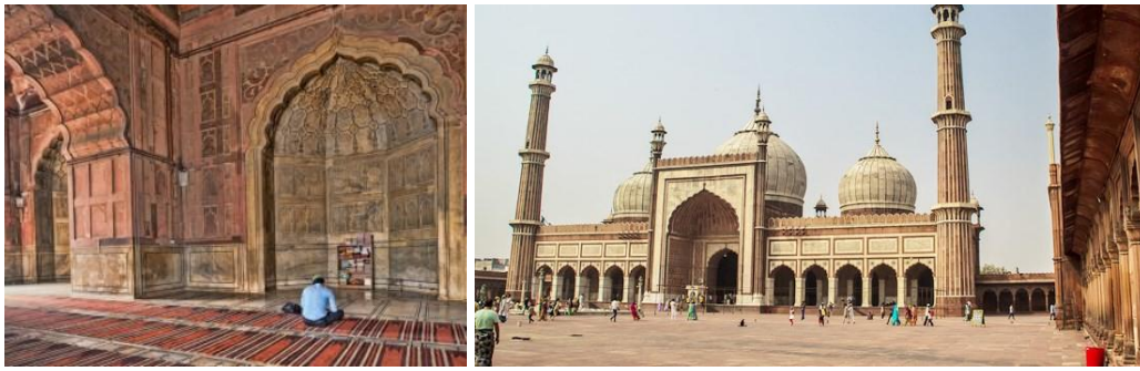
Figure 13. Double-curved shape, with a pointed or cusped top and concave curve on the inside, Jama Masjid, Delhi
