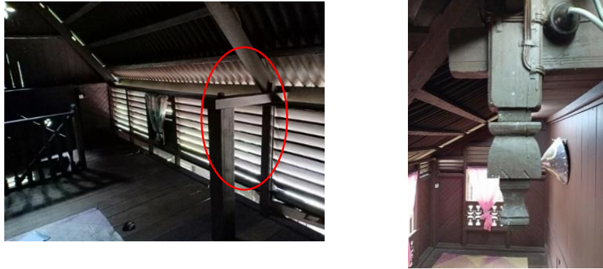
Plate 1.13 One of six tiang gantung functions as a support to roof structure that is hung in attic space (left) and One of six buah buton that was carved based on pecah empat (four broke) of tiang gantung (right) in Datuk Diwangsa's house
