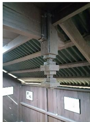
Plate 1.1 Tiang gantung in Datuk Diwangsa's house, Malay Heritage Museum, University Putra Malaysia Source: Photography by Fakhrur Razi Maamor, 2018
