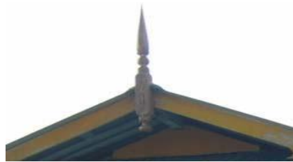
Plate 1.5 Buah buton with tapered shape that connected two pemelah long boards Source: Falsafah Seni Ukir Melayu by Azizul Azli Ahmad, 2015
