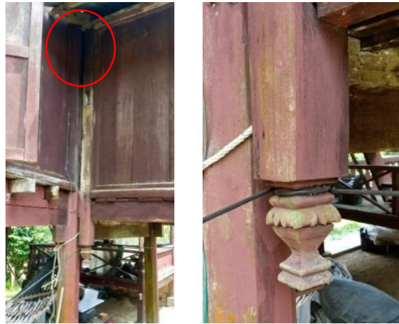
Plate 1.15 A tiang gantung on Sali's houses that serves as a supporter to long beam that goes through or penetrates the tiang gantung (left) and buah buton that is carved based on pecah empat (four broke) tiang gantung with small size (right) on Sali's house
