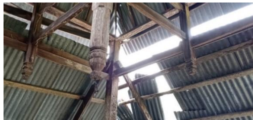
Plate 1.4 Buah buton along with tiang gantung at Kampung Parit Istana Old Mosque in Terachi
