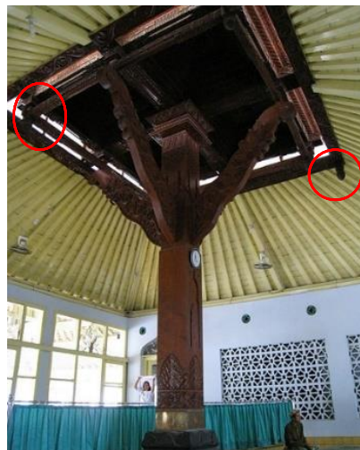
Plate 1.2 The circle shows the saka bentung with decoration at the bottom Source: Tugas Aplikom by Anggaawan, 2013
